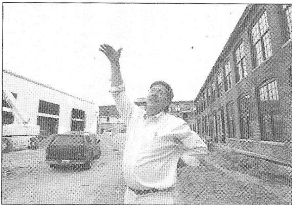
Bill Struever, president and CEO of Struever Bros. Eccles & Rouse, tours a section of the Rising Sun Mills complex being converted into a livable work space for artists in Providence. Struever Bros. is one of the developers working on a $3.1 billion master plan for downtown Yonkers.
