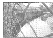
Saw Mill River: Stretches of the river that have long flowed underneath downtown would be opened.
